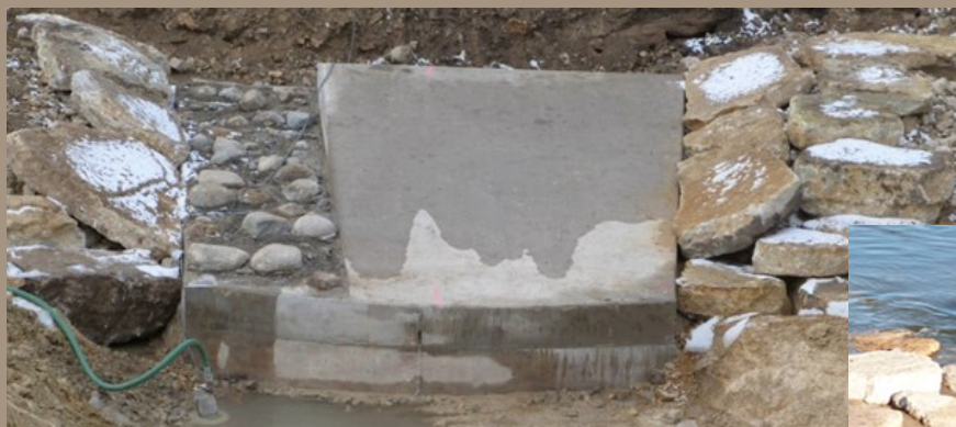
Picture 1. One of six whitewater structures after construction (top) and with flowing water (bottom). The high gradient, smooth concrete portion creates a "standing wave" for boat navigation. The fish passage channel has a more gradual slope and uses boulders to create roughness.
